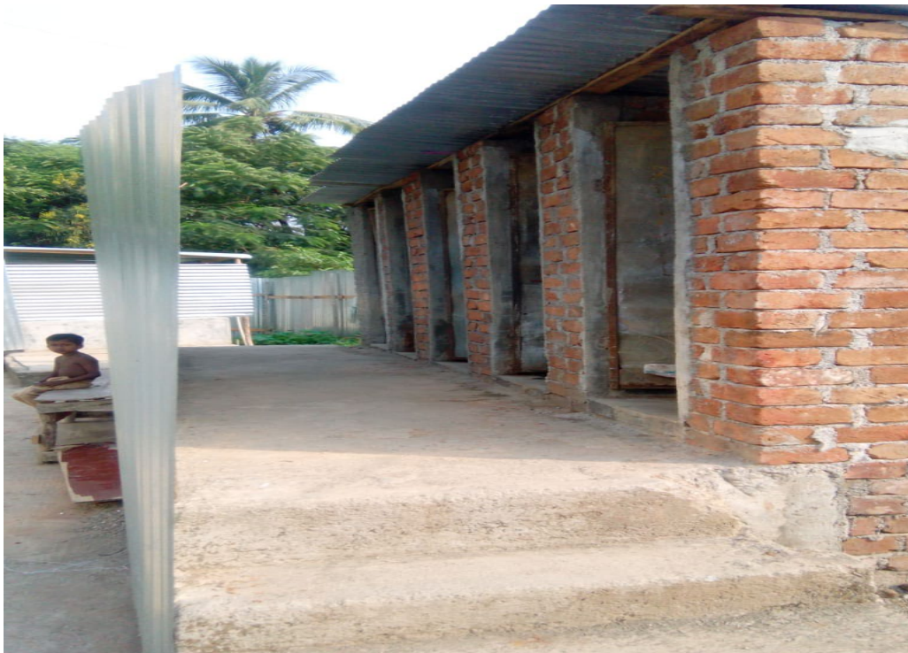
Toilet for Labours
